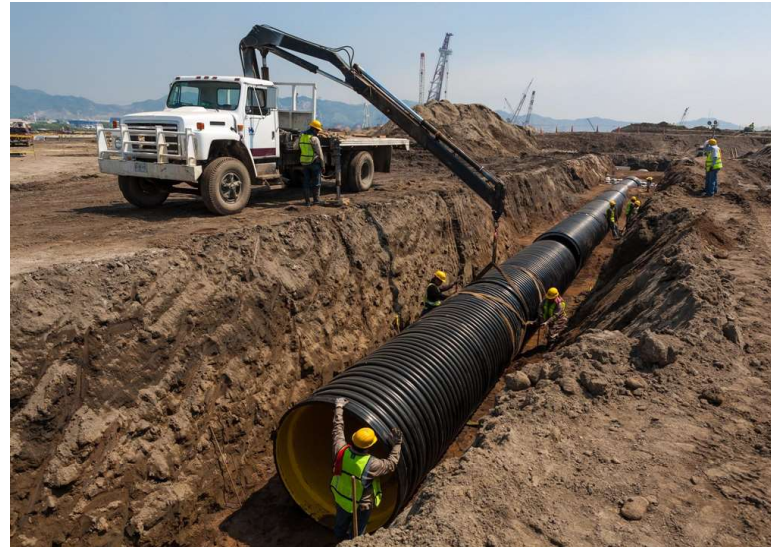
Resistant to corrosion
